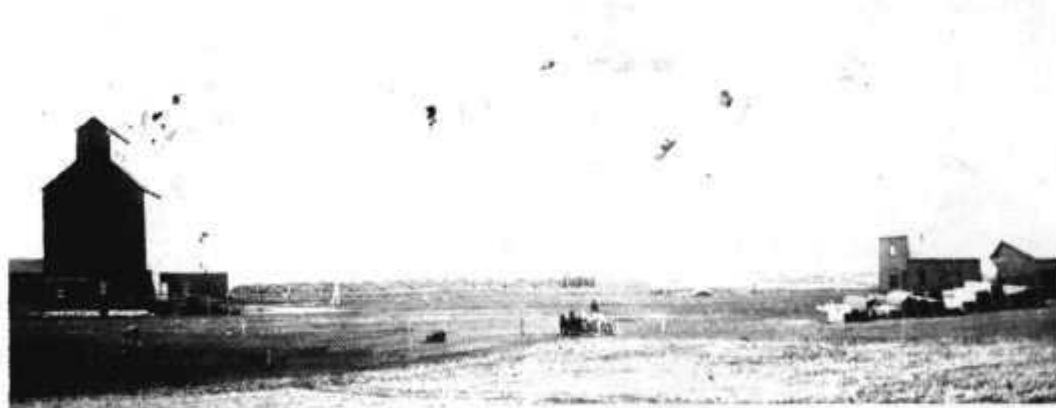
Buildings at Divide, south of Sheyenne included elevator, lumberyard and store.
