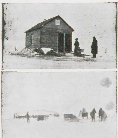
FIRST BUILDING ERECTED ON THE BOX ELDER GROVE FARM, Peter J. Leegard, Proprietor.
