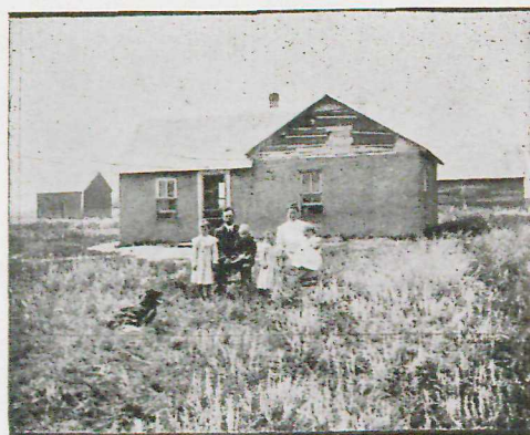
FARM BUILDINGS OF CHRIS TORNO.
