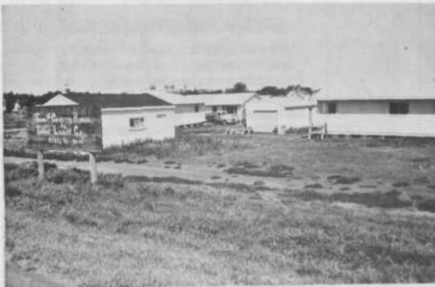
NEW HOME CONSTRUCTION
