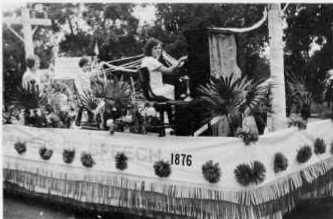
Trail County Telephone Company float with Grace Matchke at the switchboard and R. Wiseth on the left.
