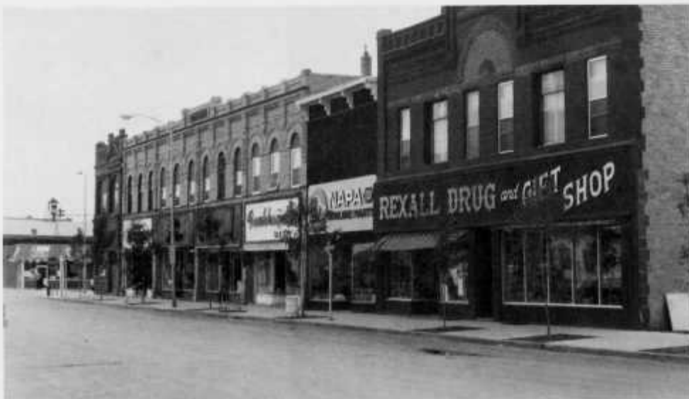
Looking east on Caledonia Avenue.
