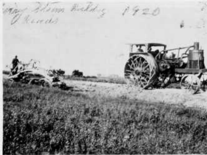
Henry Strom's road building outfit, 1920.
