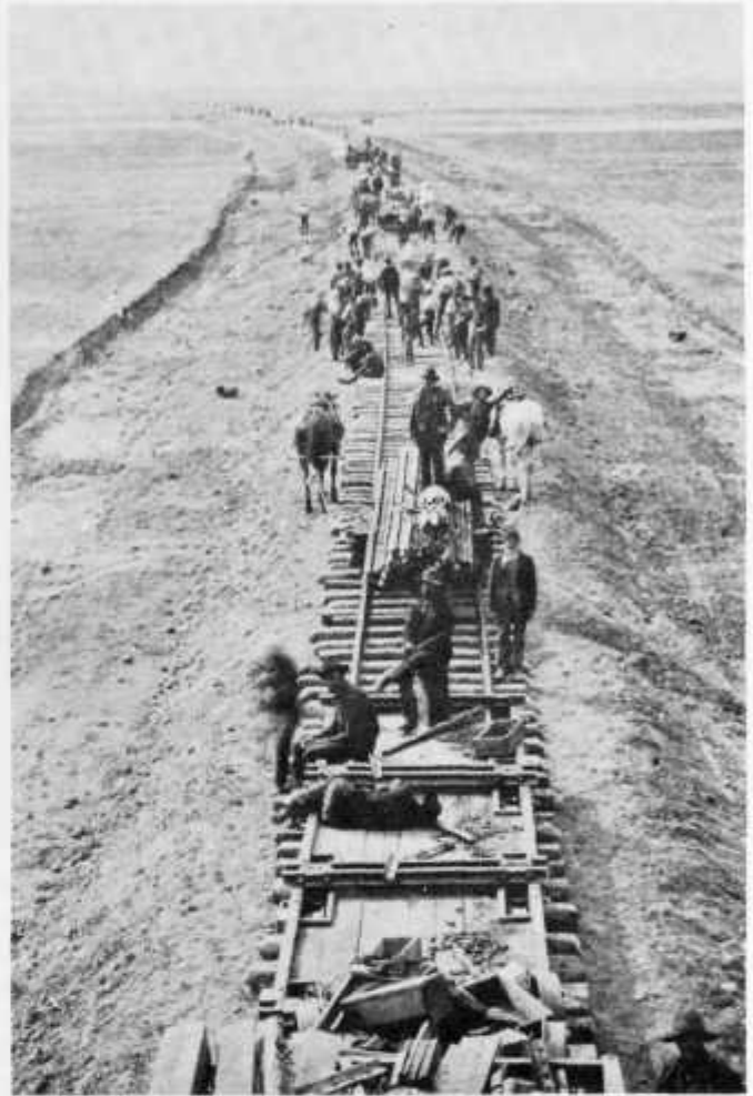
Railroad construction in Dakota.
