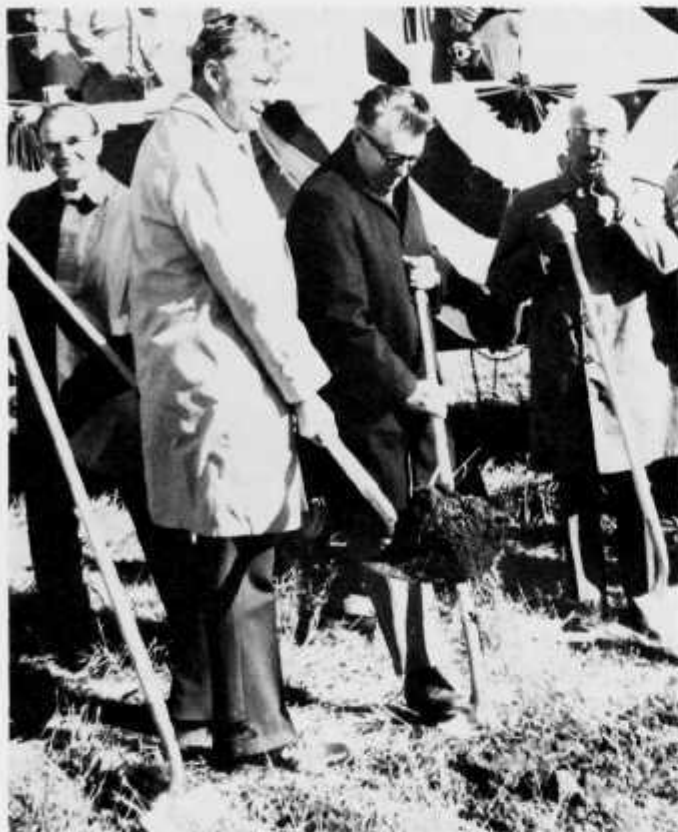
Mayor Ronald Stuart, City Auditor John Nelson, and Orin Shelley, Representative of the Bank for Cooperatives taking part in the ground breaking ceremony on Sept. 21, 1972 for the Red River Cooperative Sugar Beet Factory. U.S. Rep. Arthur Link in the background.
