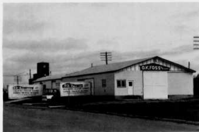
O.K. Foss Insulation & Roofing Company.
