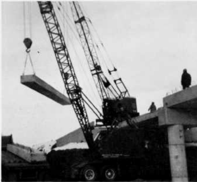
Putting up new bridge.
