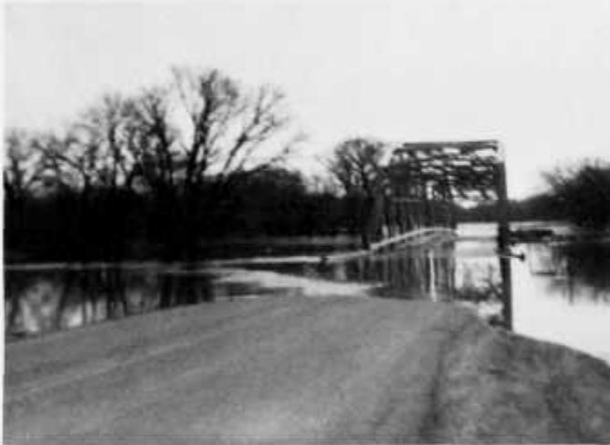
New Bridge during 1969 flood.
