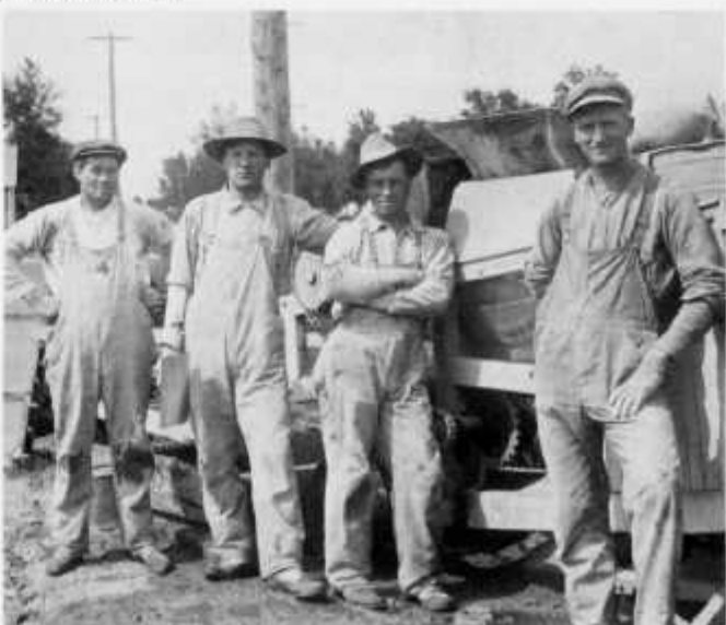
J.B. Hanson, Arne Klemetson, and Albert Anderson pouring cement in the 30's.
