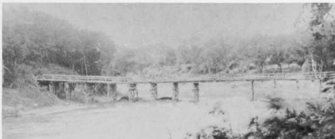
The first bridge across the Red River between Frog Point, N.D. and Climax, Minn.
