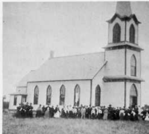
Ringsaker Church Destroyed
